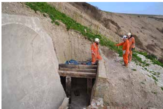
Mining engineers looking at the excavated entrance to the shelter adjacent to the 15' sound mirror. Photo Jon Barker
